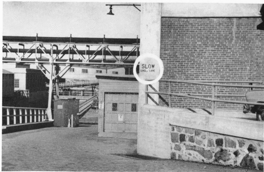
This picture shows one of the traffic hazard signs placed around the plant. Because the plant was laid out many years ago there are places where caution is necessary to avoid accidents.
